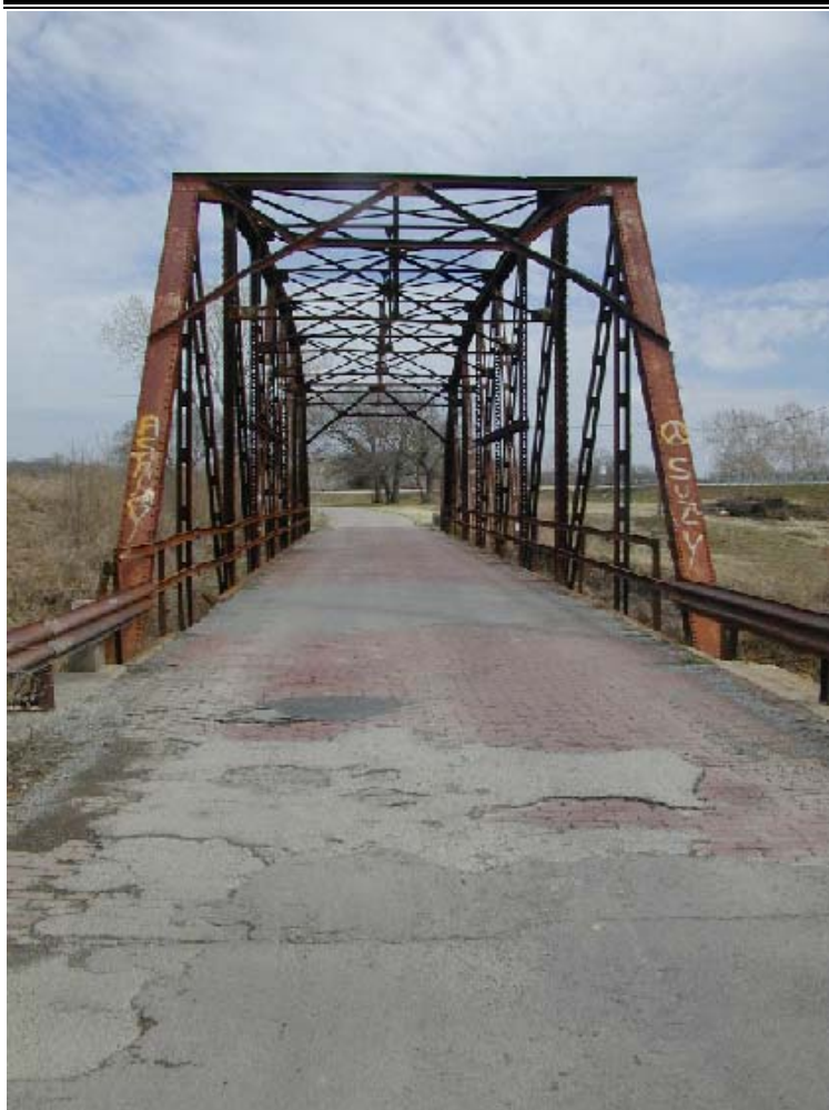
Rock Creek Bridge near Sapulpa, Oklahoma, with its brick deck, was one of the multitude of Federal Aid Projects undertaken prior to the designation of U.S. 66. Photo: Michael Cassity
