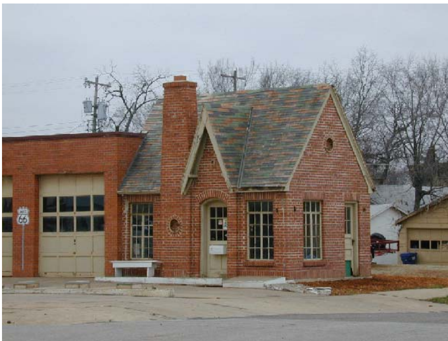
Phillips 66 Station, Chandler, Oklahoma (1930). One of Phillips' many cottage stations, this building conformed to the branded pattern of the company with its Tudor-revival connotations, its chimney, windows, and orange and blue shingles. Note the roundel for the Phillips 66 logo in the chimney and in the right gable. The two service bays at left were added during the period of historic significance as the station added service functions to gasoline sales. Photo: Michael Cassity, 2002.
