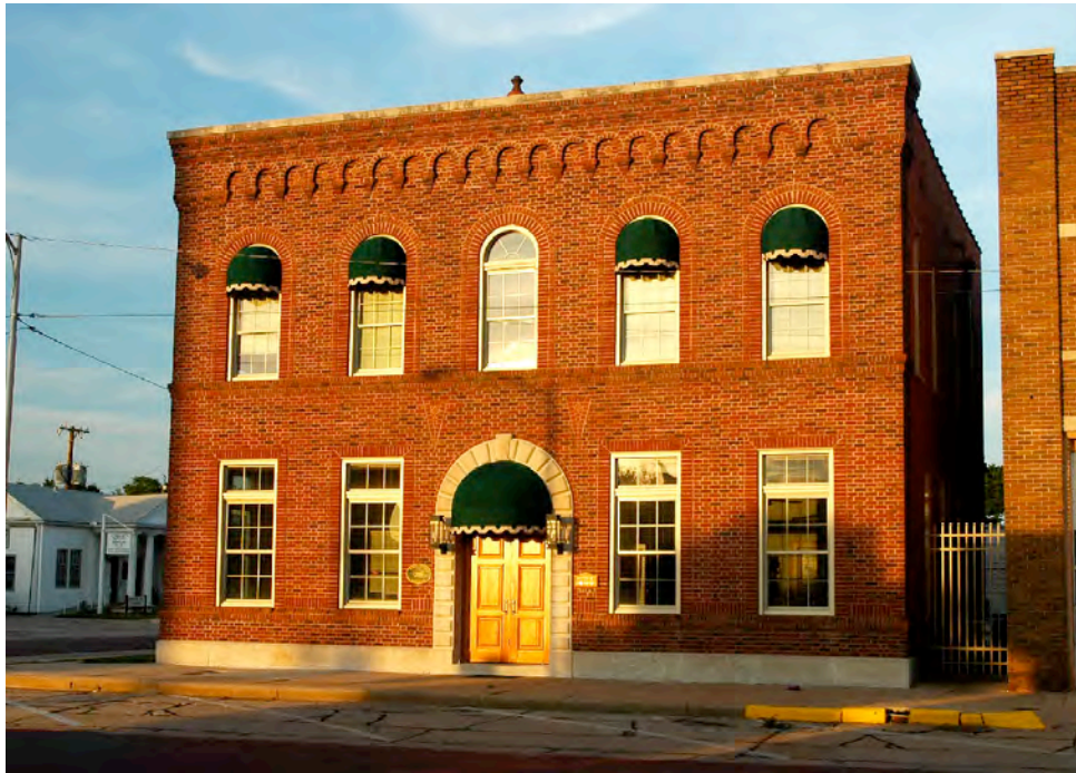
Southwest Bell Telephone Company Building, Ponca City, Oklahoma. Photo: Michael Cassity, 2008.
