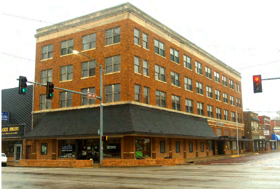
Community Building, Ponca City, Oklahoma. Photo: Michael Cassity, 2008.
