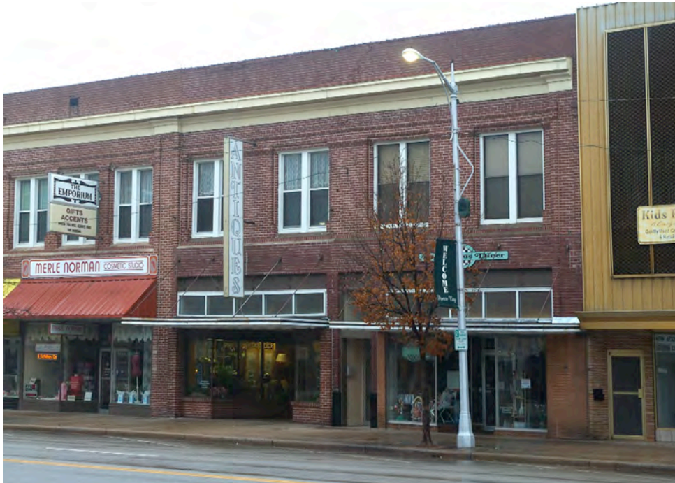
Hutchins and Hanley Building, Ponca City, Oklahoma. Photo: Michael Cassity, 2008.
