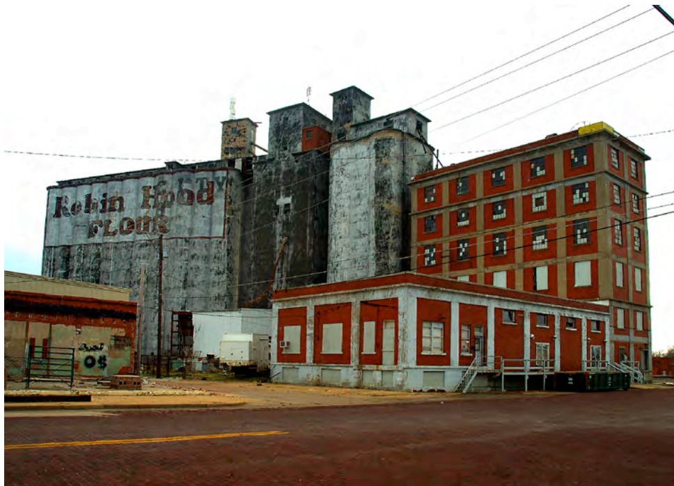
Ponca City Milling Company Elevator, Ponca City, Oklahoma. Photo: Michael Cassity, 2008.
