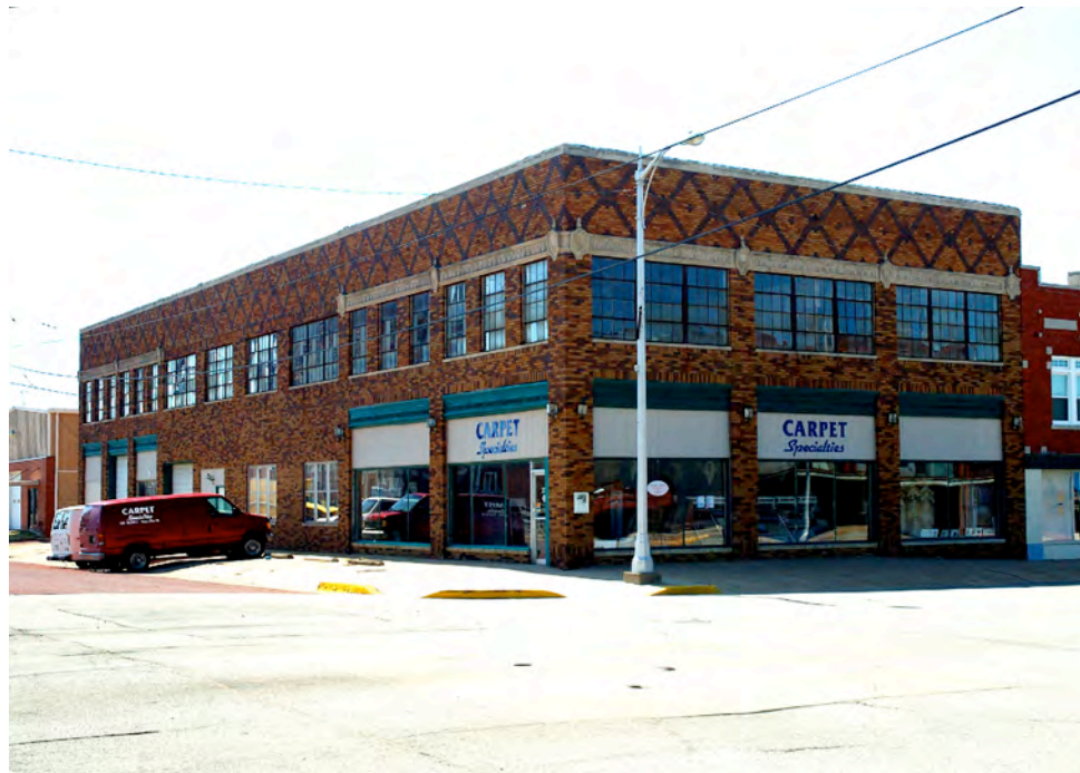
Orville Savage Motor Company Building, Ponca City, Oklahoma. Photo: Michael Cassity, 2008.
