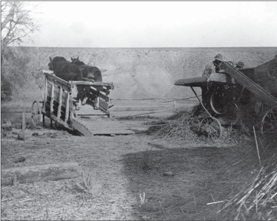
Horses on treadmill powering thresher on East Fork of Wind River. Photo: courtesy of Riverton Museum.
